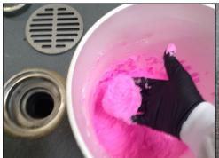
Rinse drain free of product or wash drain prior to applying Barrier FS. Remove the drain cover and use a designated glove to apply a small amount of paste to drain surfaces.
