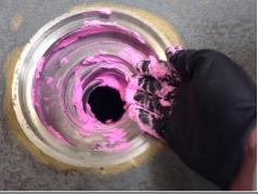
The application of paste by hand allows for the treatment paste to be forced into small spaces, under drain ledges and around drain openings reducing product and water accumulation.
