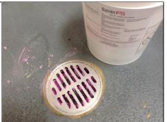
Barrier FS is a quat based cleaning compound that will physically reduce the accumulation of product, water and other processing debris in drain and floor voids. The bright color allows easy identification and ease in monitoring for determining reapplication frequency.
