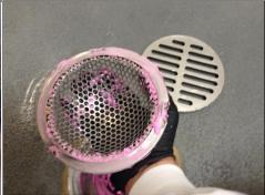
The drain screens should be lightly scrubbed with the paste so that a small amount of paste is visual. This will help identify how much water has passed over the screen between cleanings.
