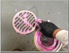
The bottom side of the drain grate should have a thin layer of paste applied to it. This will reduce the amount of product or possible build up from occurring on the underside of the grate.
