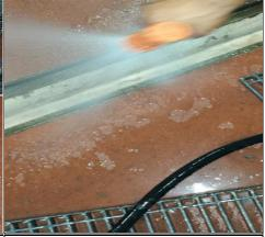
Rinse the drain with the low pressure "wide-spray pattern" nozzle to prevent over spray of debris from the drains.
