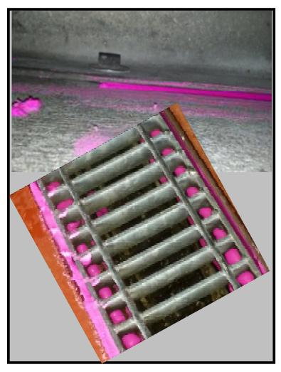
**Directions for Use:** Barrier FS should be spread into the cracks, holes and voids with tools dedicated for each specific surface type (i.e. Floors, walls, drains or structure). Apply in a uniform fashion, filling the cracks, holes or voids with the "pink paste".
