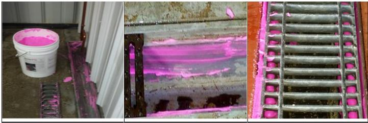
Sanitize with 400-800 ppm's of the quat sanitizer, allow excess water to dry or drain, then apply the Barrier FS paste directly.
