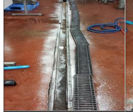
Remove drains and rinse any product to drain openings. Foam all surfaces with chlorinated alkaline foam.
