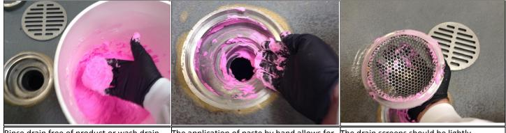
Rinse drain free of product or wash drain prior to applying Barrier FS. Remove the drain cover and use a designated glove to apply a small amount of paste to drain surfaces.
